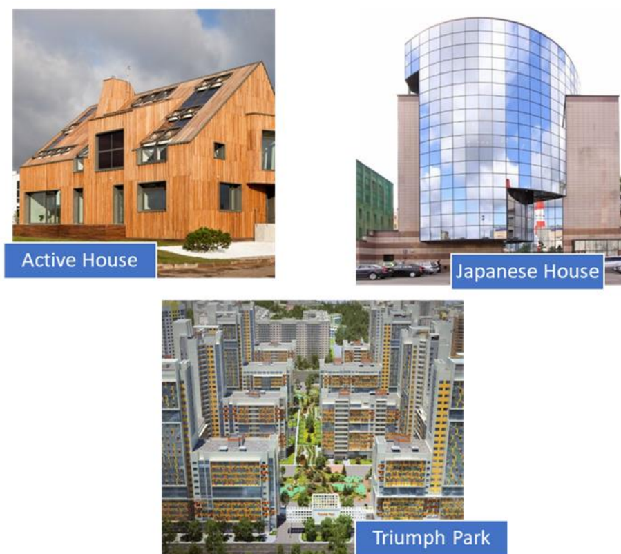
Fig. 6. Buildings using green technologies in Russia.
