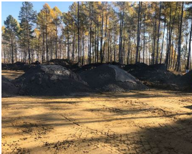
Fig. 2. Erection of earth bed layers from ash and slag mixture.
