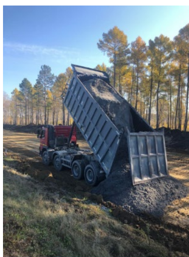
Fig. 3. Erection of earth bed layers from ash and slag mixture.
