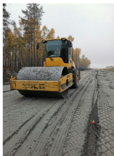
Fig. 3. Erection of earth bed layers from ash and slag mixture.
